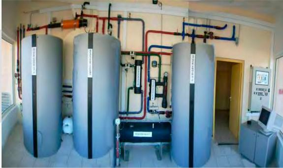
Figure 3a :  $\text{BaCl}_2/\text{NH}_3$  thermochemical process coupled to  $20\text{m}^2$  of flat plate solar collectors for solar air-conditioning
